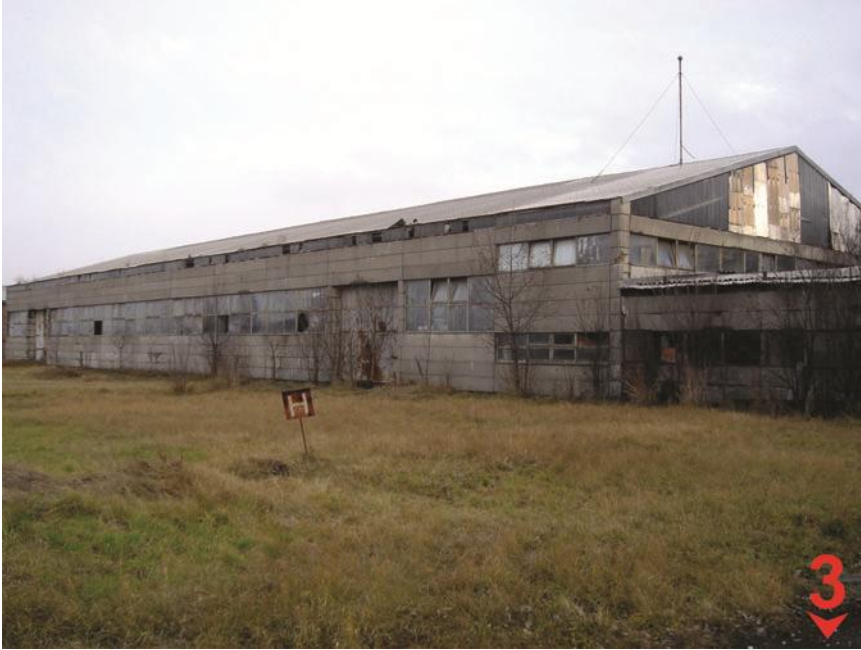
Photo 36- Existing administration offices (self-made).
