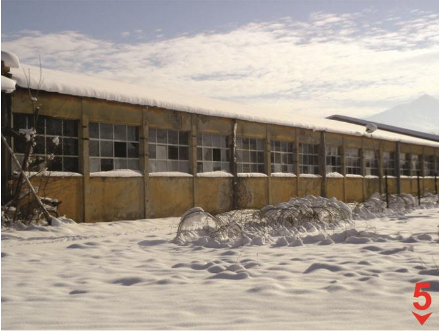
Photo 38- Existing part of the factory complex (self-made)
