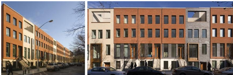
Photo 19- Brooklyn (New York), the State Street Townhouses are a continuous row of new, single-family townhouses where the architect depicts repetition and variations on the design theme (source demel.net/statestreet).
