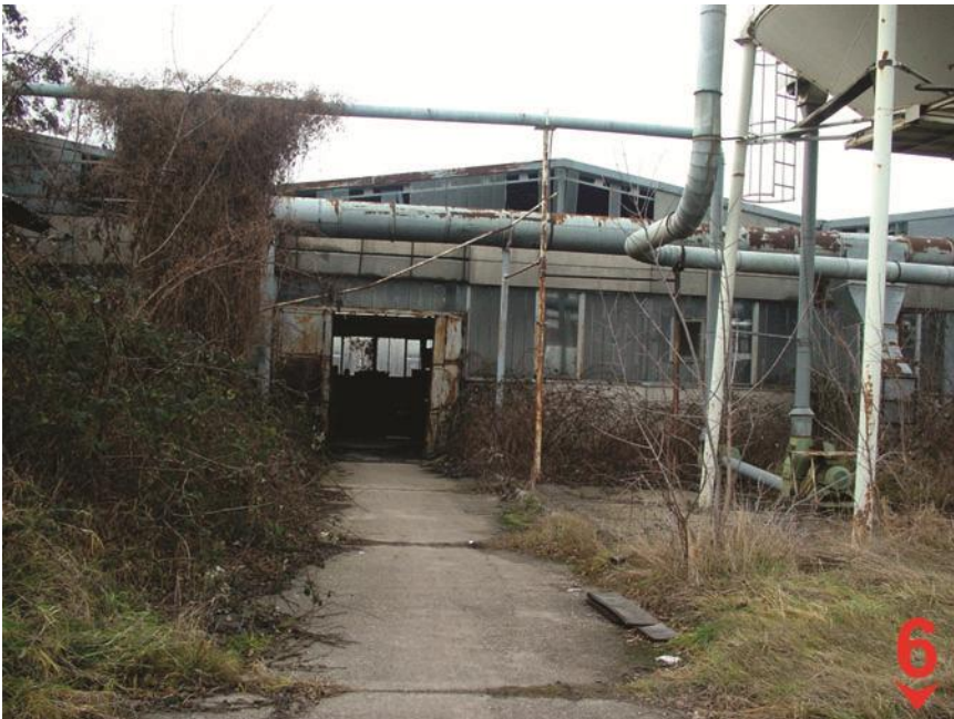
Photo 39- Existing part of the factory complex (self-made)
