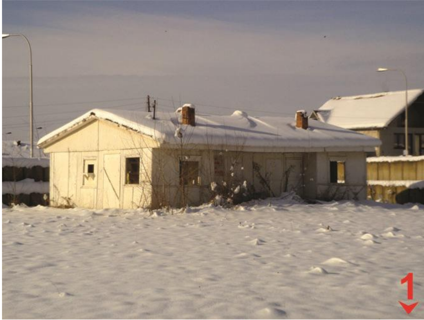
Photo 34- Existing administration offices (self-made)
