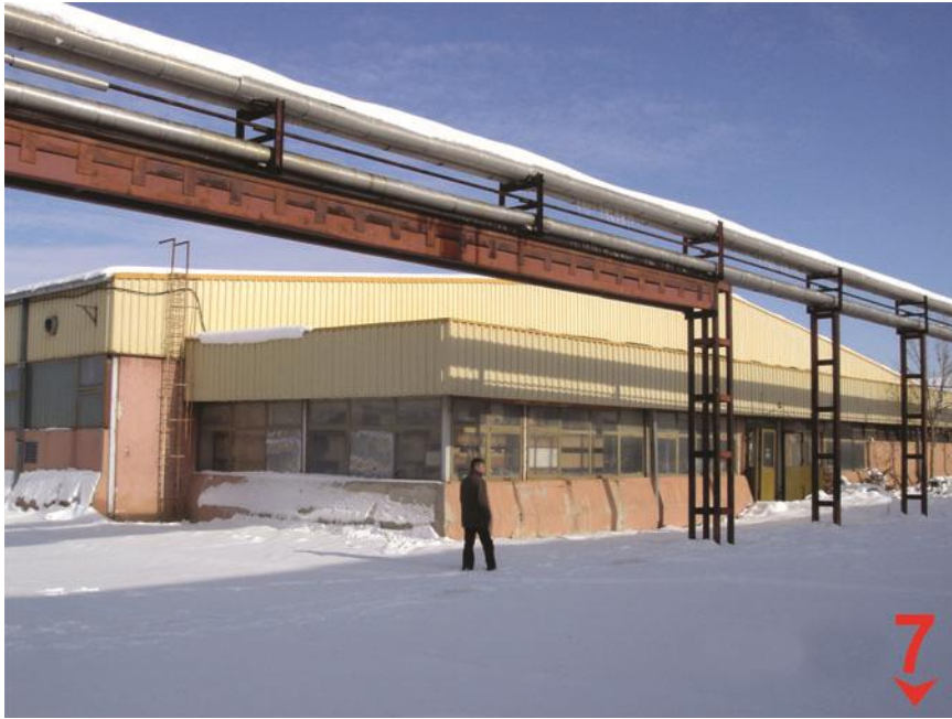
Photo 40- Existing part of the factory complex (self-made)
