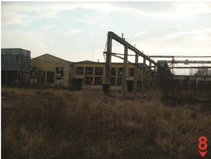
Photo 41- Existing part of the factory complex (self-made)
